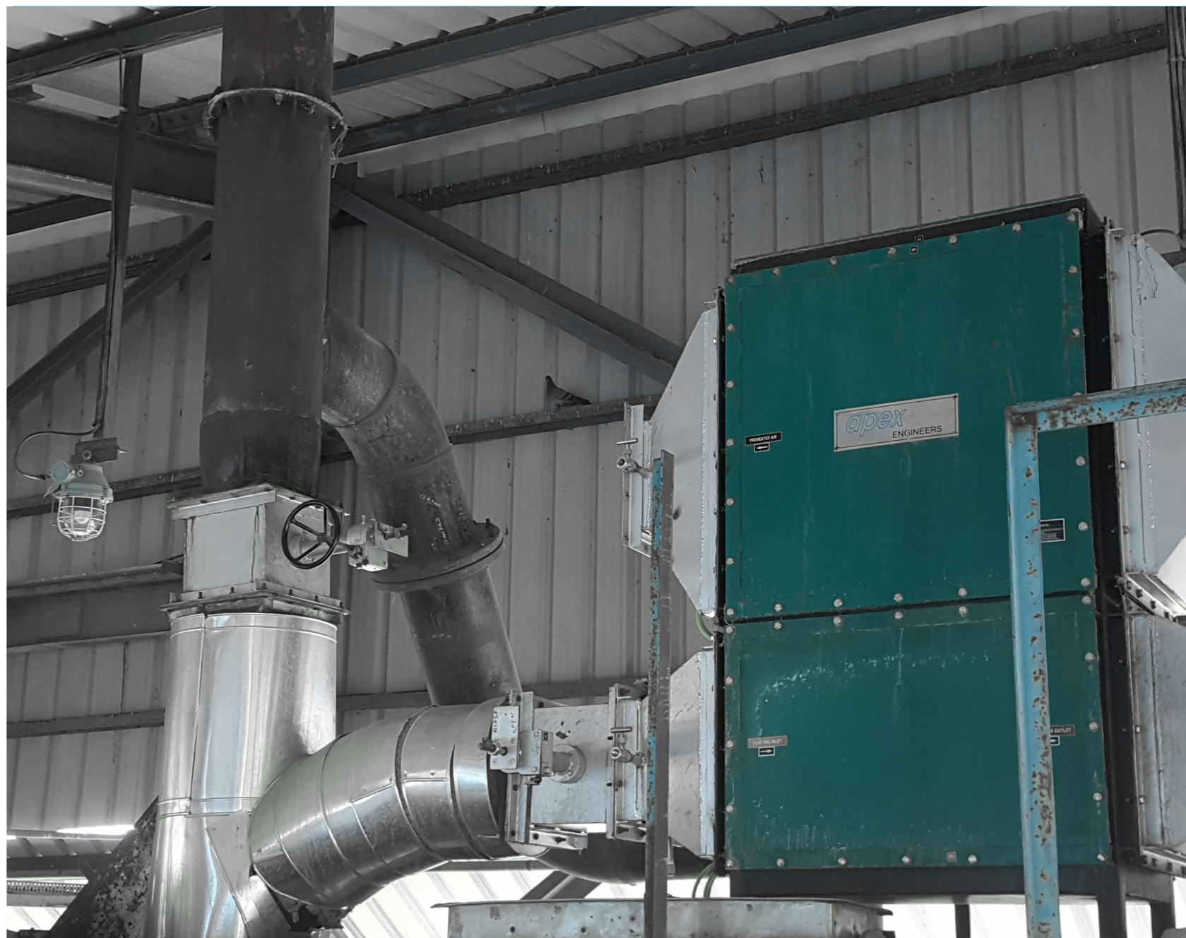
Heat pipe at our Valia Plant's spray drier unit that helps us save over 60,000 m 3 of natural gas per annum
